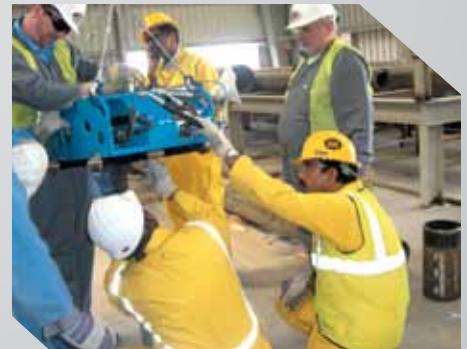
Cold Cutting Machine Installation
